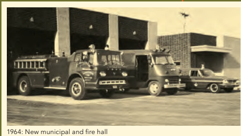
1964: New municipal and fire hall
